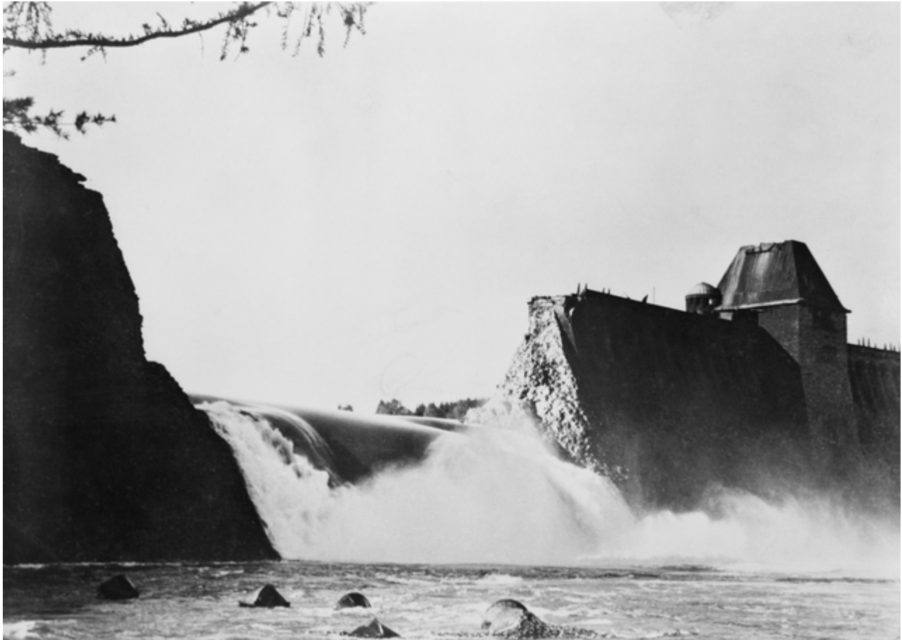
Mohne Dam breached with water cascading down the valley on the 17 May 1943 after the spectacular attack the night before by 617 SQN.(AWM)
